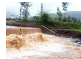
Check dam at Nashik
